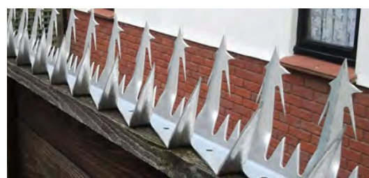
Wall spikes used on wood fence
